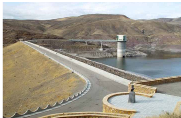
Figure 1 | Sattarkhan earthfill dam.
