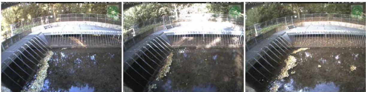
Figure 6 | Samples of images wrongly detected as blocked by the classifier and the Siamese network at the Barnstaple location.
