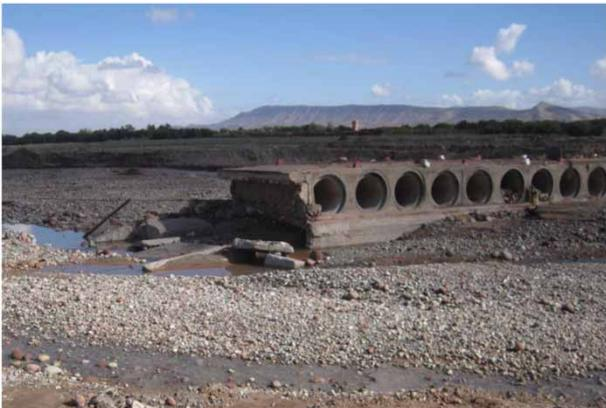
**Figure 7** | Part of Zat bridge washed away by the November 2014 flood (source: Tensift Hydraulic Basin Agency).
