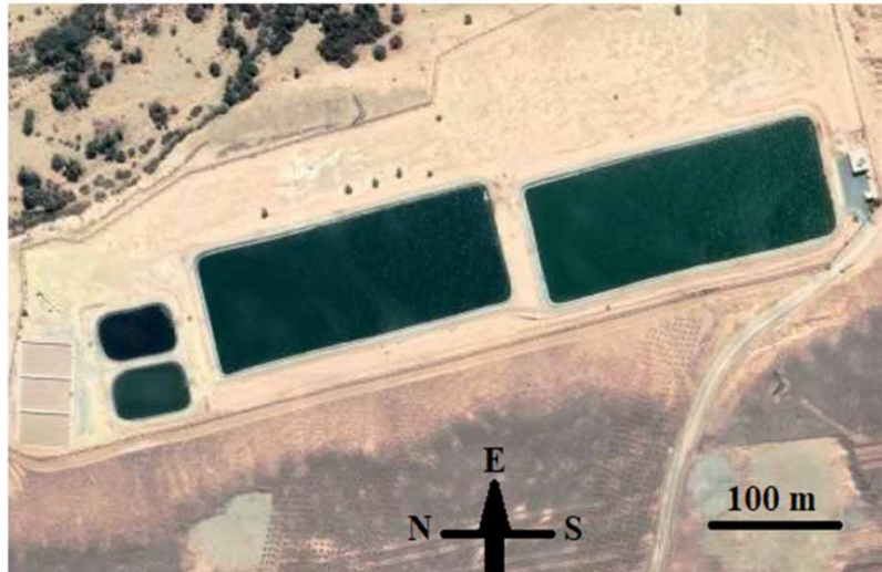
Figure 2 | Satellite picture of Assa's current WWTP.
