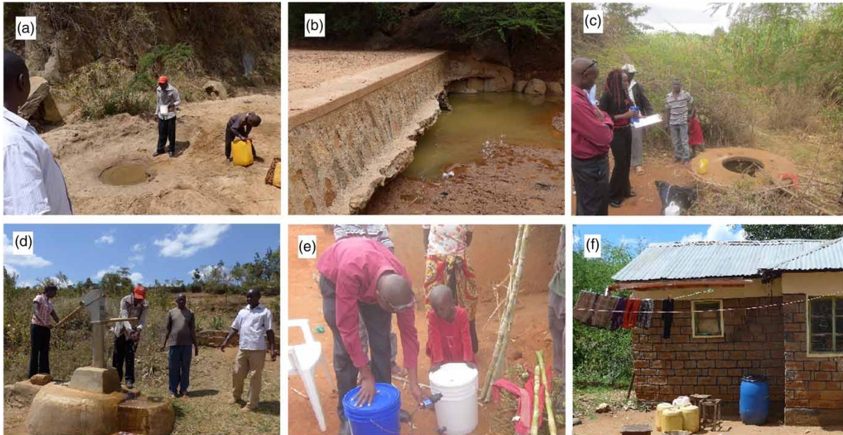
Figure 1 | Examples from categories of water sources at sand dams used for this study: (a) scoop hole, (b) surface water below the eroded dam, (c) hand dug well, (d) pump well adjacent to sand dam, (e) household water container and (f) rain barrel (blue) for roof water collection. Please refer to the online version of this paper to see this figure in color: http://doi.org/10.2166/wh.2020.192 .
