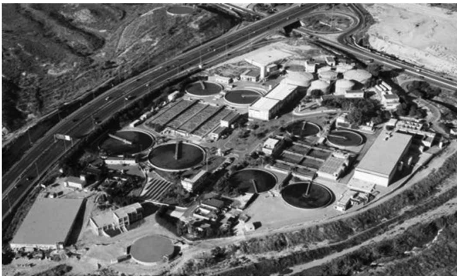
Figure 1 | Rincón de León WWTP-WRP (EPSAR).
