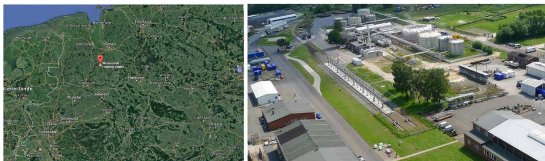
Figure 2 | Main treatment facility of the oil field Barnstorf in Lower Saxony, Germany (source: Google, Wintershall Dea).
