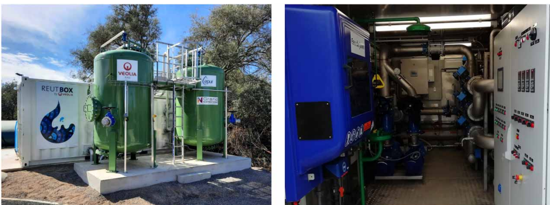
Figure 4 | Pictures of a standard containerised 10 \text{m}^3/\text{h} REUT box.
