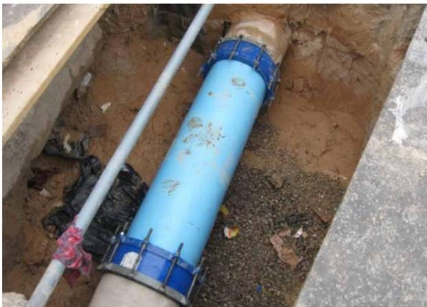
**Figure 5** | Lined pipe sections connected by PVC pipe (with permission from Matthews *et al.* 2015).
