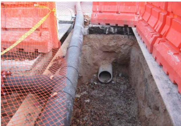
**Figure 2** | Access pit with pipe removed (right) and bypass (left) (with permission from Matthews *et al.* 2015).
