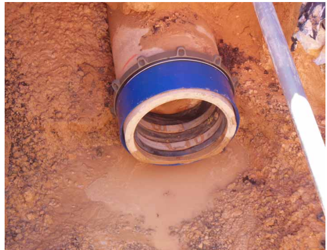
Figure 4 | Finished end seal.
