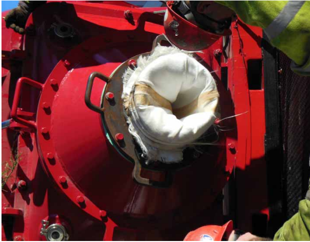
Figure 2 | Inverted liner end attached to pressure vessel opening.
