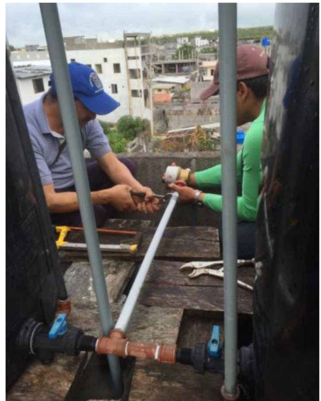
Figure 1 | Installation of water meters.
