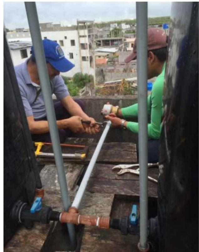
Figure 1 | Installation of water meters.
