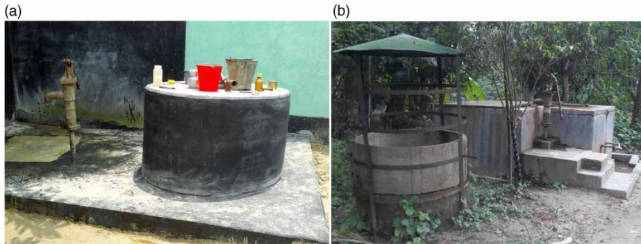
Figure 2 | Photographs of typical dug wells in the study area: (a) GO-installed dug well with hand tube well and (b) NGO-installed dug well with a slow sand filtration system.
