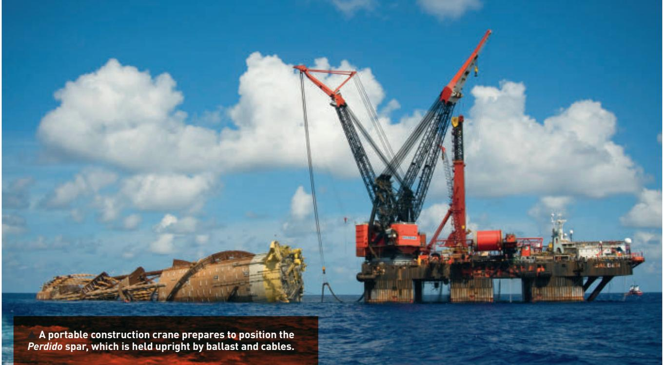
A portable construction crane prepares to position the *Perdido* spar, which is held upright by ballast and cables.
