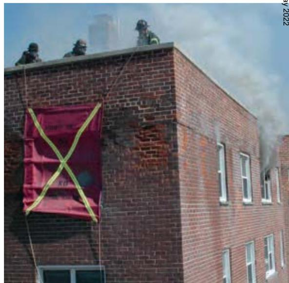
experiments demonstrated that wind control devices and high-rise nozzle deployment were effective in reducing the thermal hazard in the corridor. However, firefighters do not fight fires in laboratories; thus the next step was to have firefighters employ the new tactics in live-burn experiments.
