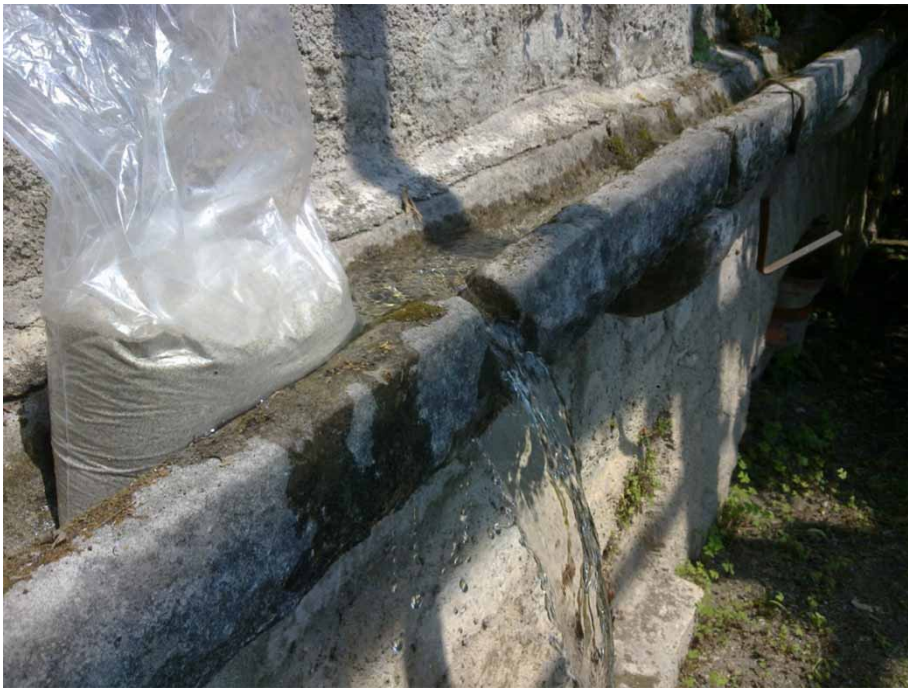
Figure 6 | Ancient distribution system in a lemon garden at Lake Garda (Alto Garda Bresciano, Italy). The spilling water was originally accompanied to the bottom of the tree in order to prevent excavation.
