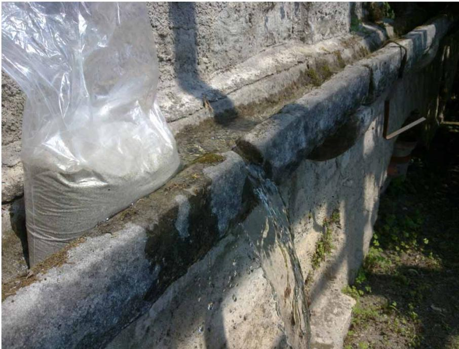
**Figure 6** | Ancient distribution system in a lemon garden at Lake Garda (Alto Garda Bresciano, Italy). The spilling water was originally accompanied to the bottom of the tree in order to prevent excavation.
