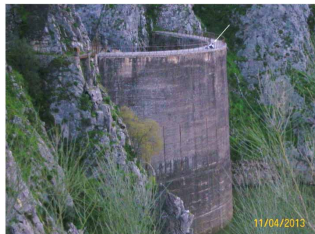
Figure 2 | Current view of the Montejaque dam.
