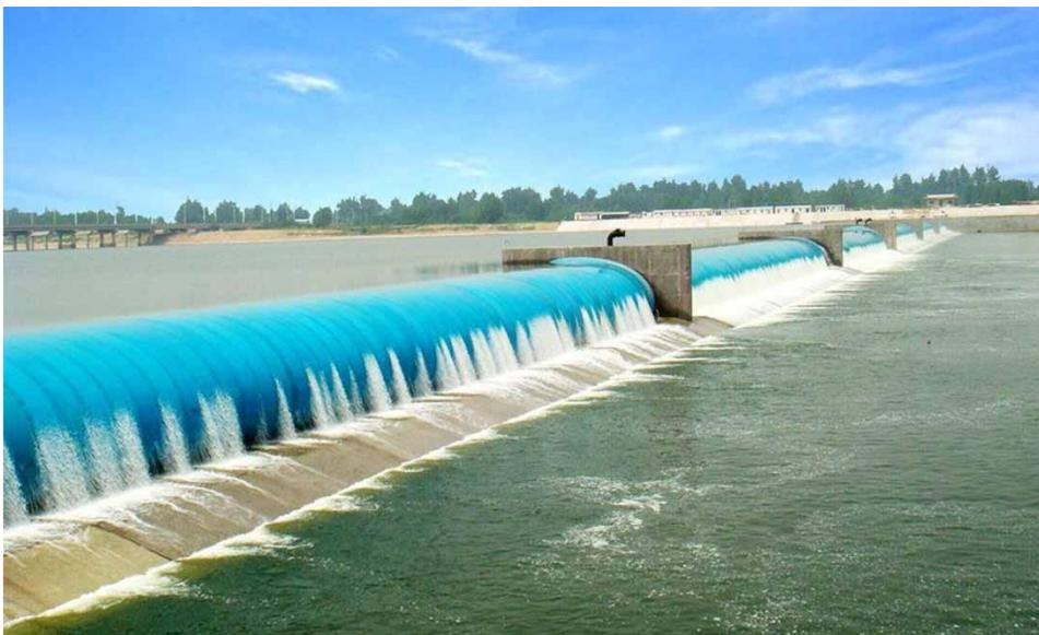
**Figure 1** | The rubber dam project in Bahe River.
