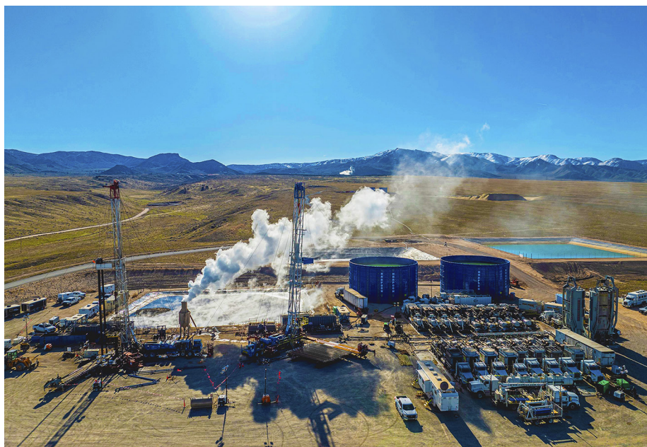
Figure 1. A view of the Utah FORGE geothermal site and operations during groundbreaking April 2024 EGS stimulation and circulation. Photo courtesy of Utah FORGE and Eric Larson (Flash Point SLC).
