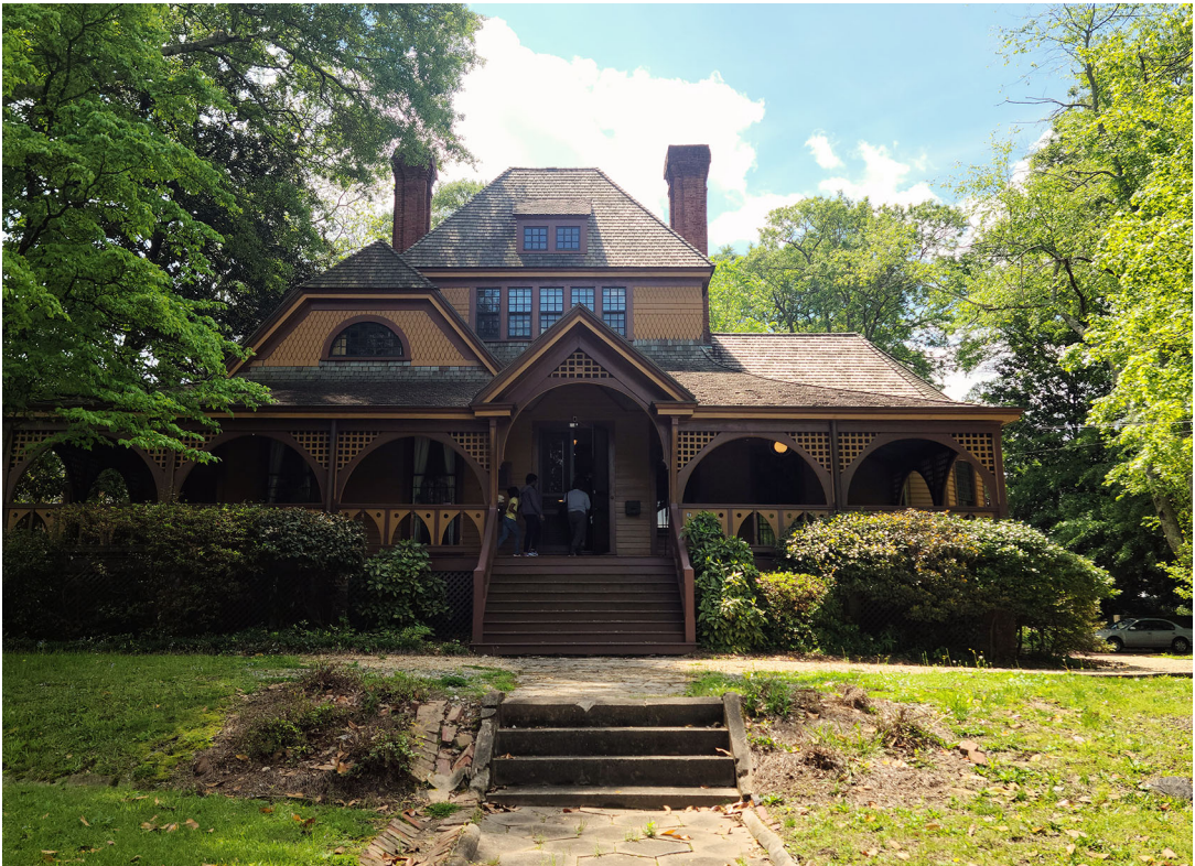
Exterior, The Wren's Nest, in the West End Neighborhood of Atlanta, Georgia. Built circa 1870 as a farmhouse; journalist and author Joel Chandler Harris paid for an expansion and Queen Anne style renovation in the 1880s. The house became a National Historic Landmark in 1962. (Photograph by author)
