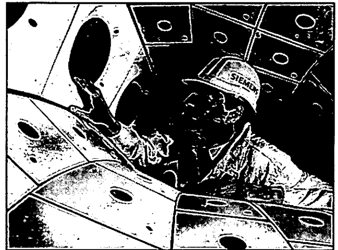
Figure 8. Inspection of Burner in HBR™ Combustor
