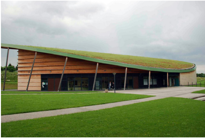
Fig. 3. New applications for growing media are rapidly emerging, such as for green roofs, urban and space agriculture, and waste filters. (Photo by Sylvain Charpentier showing a green roof on a gymnasium in Angers, France.)
