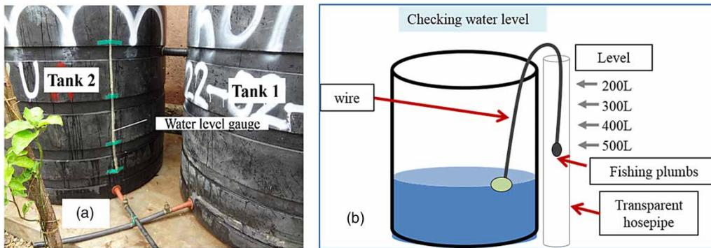
**Figure 4** | (a) Water level gauge taped onto the supply Tank 2 and (b) illustrations of water level monitoring with the gauge.
