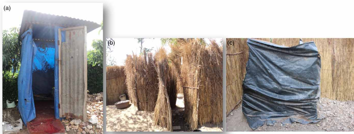
Figure 1 | Typical Shackleton pit latrines (a) covered with a mixture of iron sheets and tent made of tarpaulin material, (b) covered with thatching grass and (c) covered with a 250 µm plastic tent.
