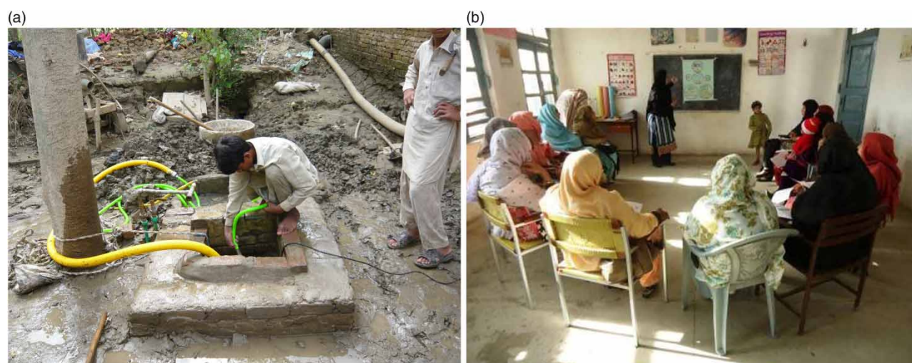
Figure 1 | (a) 'Hard component' – well cleaning and well-rehabilitation activities after WHO Technical note No. 1 on drinking-water, sanitation and hygiene in emergencies: 'Cleaning and disinfecting wells'. (b) 'Soft component' – hygiene promotion, training of teachers and school children on water and hygiene.
