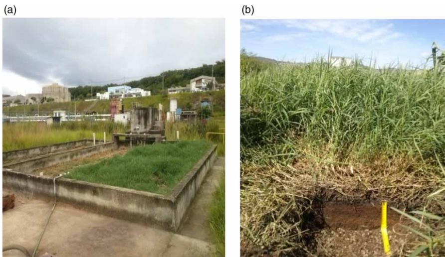
**Figure 1** | Panoramic view of the vertical flow constructed wetlands, receiver of sanitary sewage sludge from the septic tank and cultivated with tifton 85 grass (a), and detail of the profile of organic material accumulated on the substrate of the system, where samples were collected (b).
