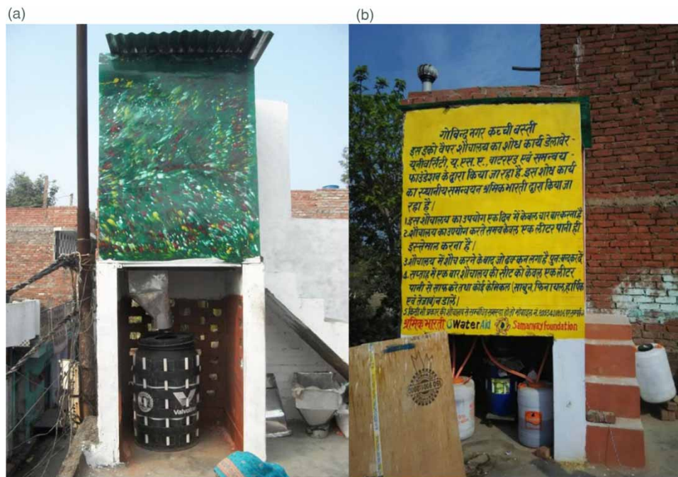
Figure 1 | EVT field setup in Kanpur, India for the (a) Year 1 field test with a laminate-lined 208 L (55 gallon) drum and (b) Year 2 field test with a laminate-lined 40 L drum and urine-diverting Eco-San pan. All toilets were fitted with a ventilation pipe with wind fan for odor control. Please refer to the online version of this paper to see this figure in colour: http://dx.doi.org/10.2166/washdev.2021.011 .
