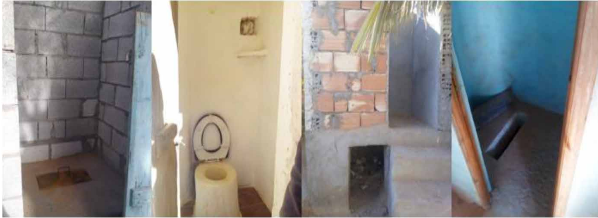
Figure 5 | New dry toilets in Beni Isguen, 2019.
