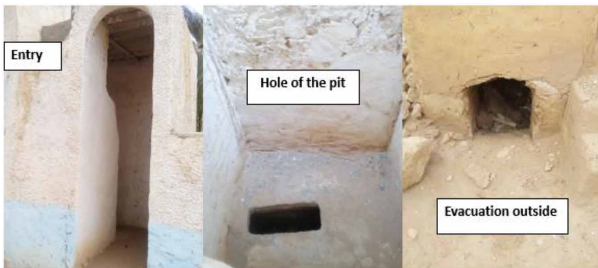
Figure 3 | Dry toilet architecture in the M'zab valley.
