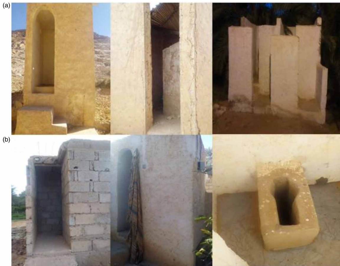
Figure 4 | Private and public dry toilets in the M'zab Valley: (a) private and (b) public.
