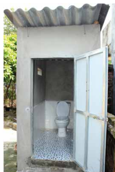
Septic Tank Latrine
