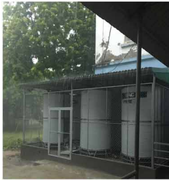
RFD (Rainwater for Drinking) System at Ly Nhan Health Care Facility, Vietnam
