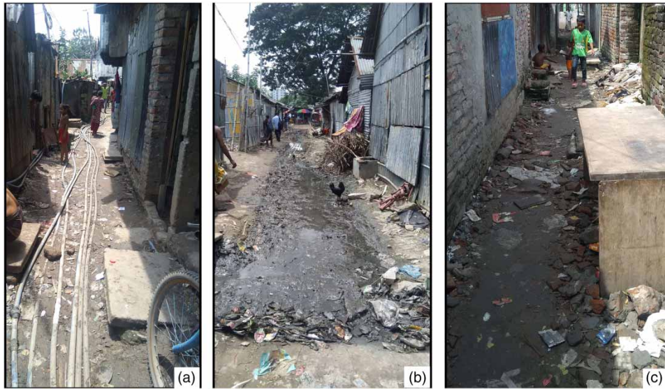
Figure 3 | Narrow communication roads in slums with (a) pipeline connections blocking road spaces, (b) slippery conditions due to mud and puddles even during dry season, and (c) filled up bricks and construction materials.
