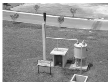
Figure 5.21. View of a hydraulic seal and gas burner (source: Ipatinga WWTP, Minas Gerais, Brazil)
