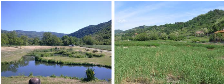
Figure 6.8 Case study 6 – Dicomano Wastewater Treatment Plant (Italy).
