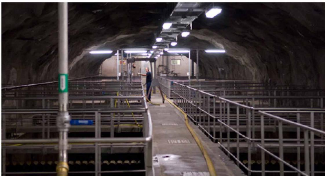
**Figure 4** | Existing secondary clarifier, view from effluent channel (showing the cavern roof at the top).
