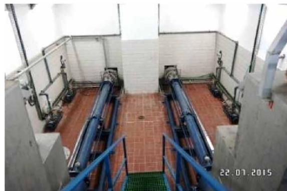
**Figure 5** | Dewatered sludge pumps.
