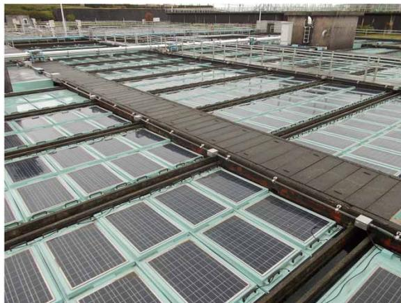
**Figure 2** | Solar power generation equipment on settling ponds at Kosuzume Purification Plant.
