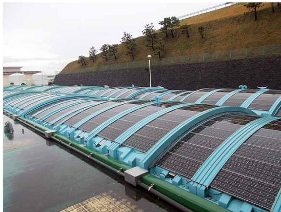
**Figure 1** | Solar power generation equipment on filtration ponds at Kosuzume Purification Plant.
