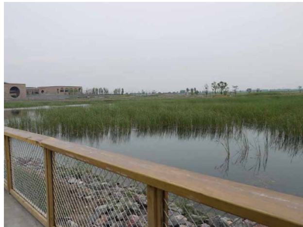
Figure 8 | One of the detention/treatment ponds in Yinchuan New Town.
