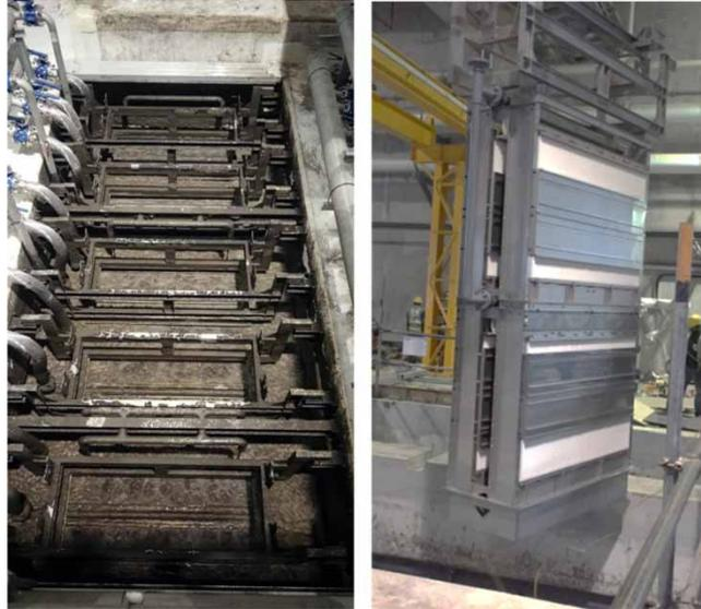
**Figure 1** | Picture of the membrane tank (left) and the membrane unit (right).
