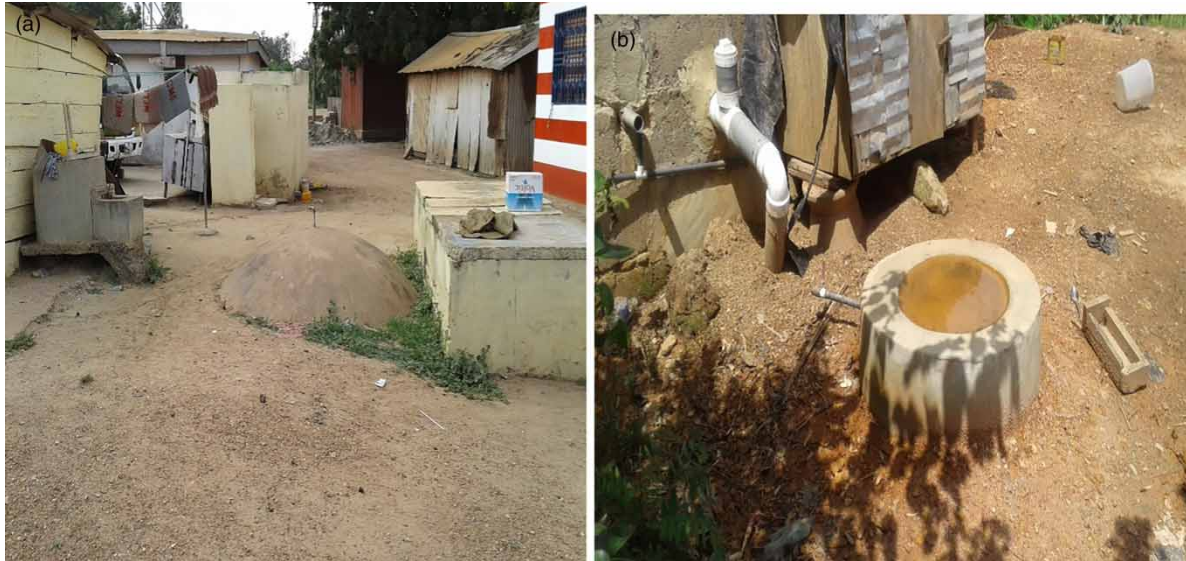
Figure 5 | (a) Remains of a fixed-dome digester at Appolonia, Accra, October 2017; (b) fixed-dome digester not connected to a kitchen at Cape Coast, Central region, October 2017.
