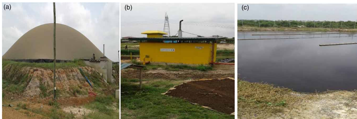
Figure 7 | (a) The Safisana fixed dome biogas plant, Ashaiman, Accra, September 2017, (b) the CHP at the Safisana Ashaiman site, September 2017; (c) Waste stabilisation pond with baffles at the Ashaiman site for treatment of liquid waste from the drying beds, September 2017.
