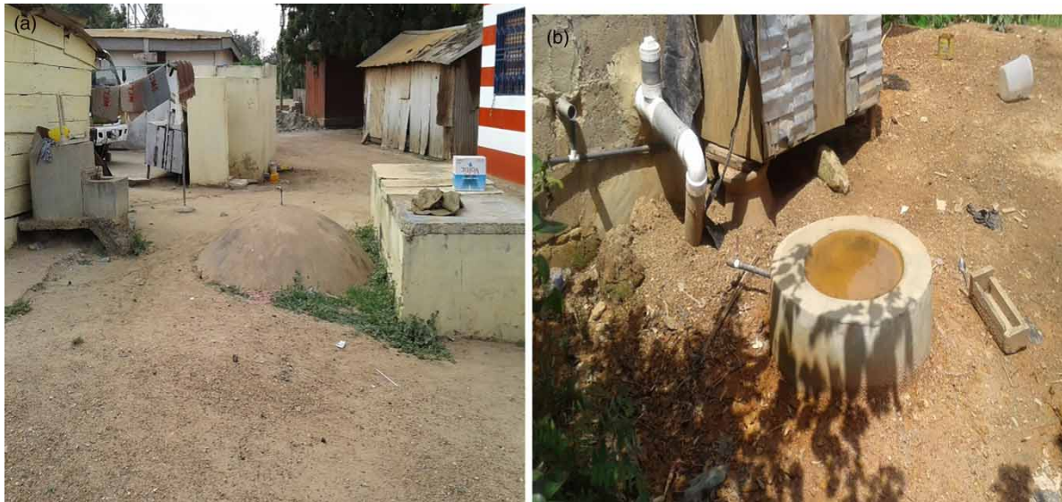
Figure 5 | (a) Remains of a fixed-dome digester at Appolonia, Accra, October 2017; (b) fixed-dome digester not connected to a kitchen at Cape Coast, Central region, October 2017.
