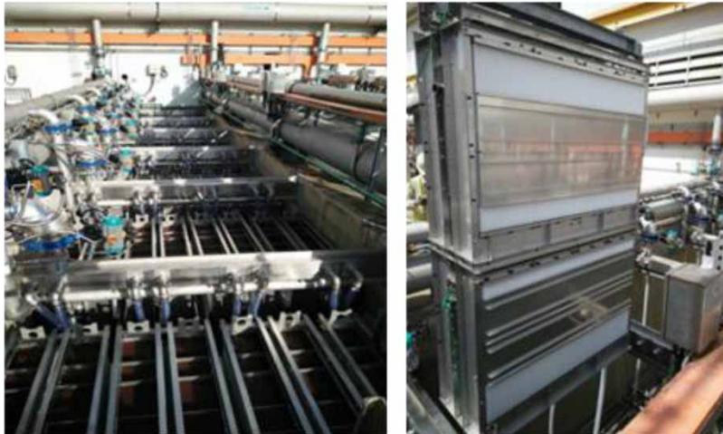
**Figure 2** | Pictures of the membrane tank (left) and the membrane unit (right) in CAWW.
