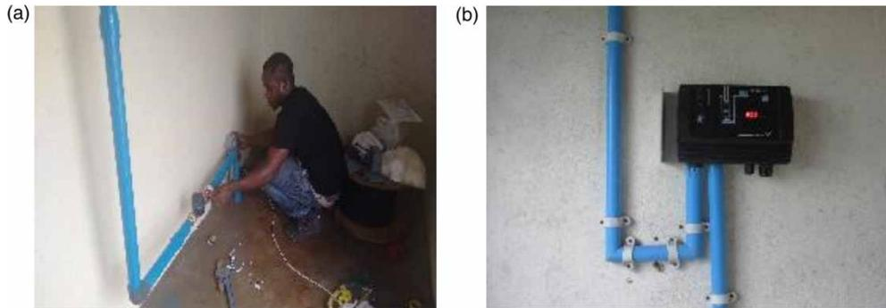
**Figure 4** | (a) Satellite water meter and communicator installation (b) CU200 as installed in the enclosure.
