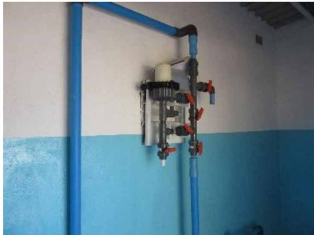
**Figure 1** | Basic Water Mission portable chlorinator.
