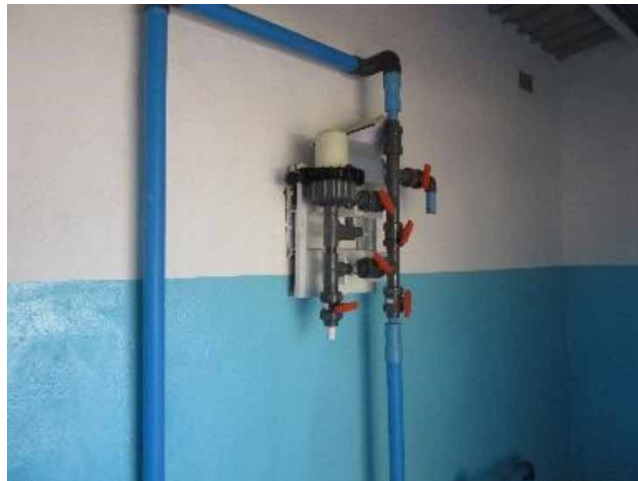
Figure 1 | Basic Water Mission portable chlorinator.
