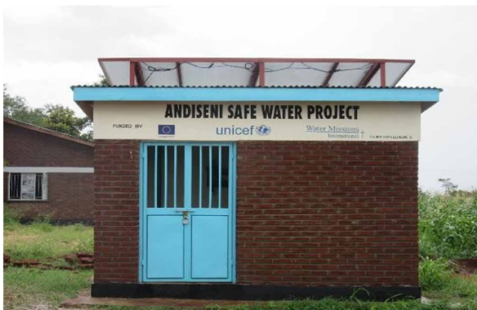
Figure 3 | A sample of a treatment and solar power house at Andiseni in Blantyre.
