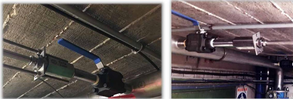
**Figure 4** | Online lead and cast iron corrosion probes at plant outlet.
