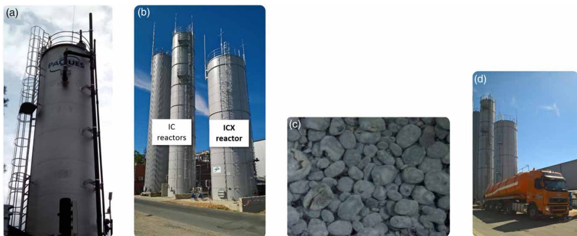
Figure 2 | Photos of the ICX demonstration reactor (a) full scale ICX installation (b), anaerobic granules cultivated in the full scale ICX reactor (c) and truck harvesting excess anaerobic granular biomass (d).
