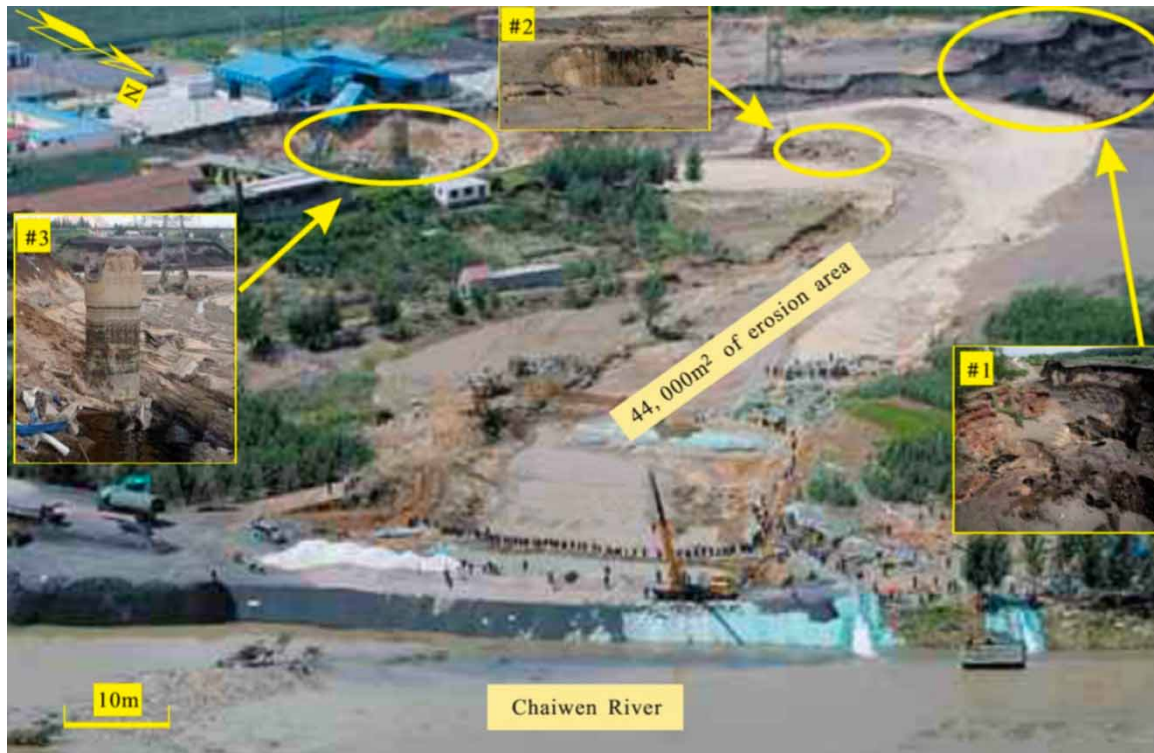
Figure 3 | Erosion area after Chaiwen levee failure (Huayuan Mining Co.).
