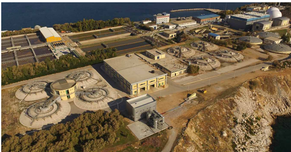
Figure 1 | Aerial view of the THP plant (bottom) and 8 mesophilic anaerobic digesters at Psyttalia WWTP.
