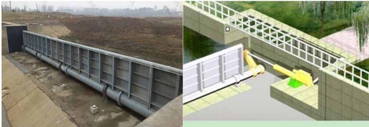
Figure 1 | Bottom shaft driving flap gate schematic diagram.
