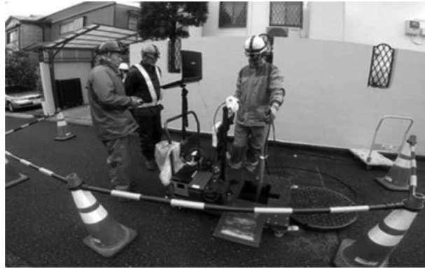
Figure 4 | Operators working from above ground in UAV inspection.
